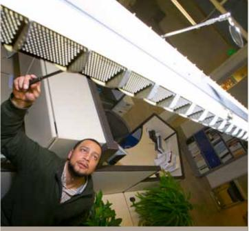
Left, Brower uses a ballast discriminator to determine the efficiency of a lighting fixture. Above, he uses a mirror to check the wattage of a lamp.
